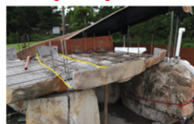
5. Place Grotto Lids, cut as needed. Splice steel. Brace.
