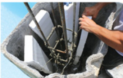
4. Fill with 3000 psi concrete mix. Foam can be used as filler.
