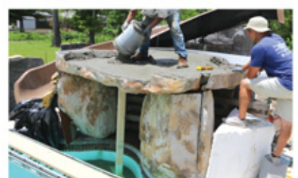
6. Top requires 1 yard of concrete. Note T brace under front grotto.
