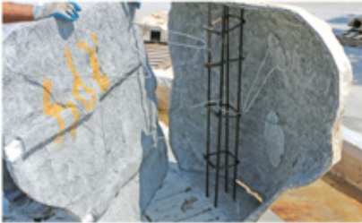
1. Columns are clam shell pieces wired to a rebar column, part of kit.
