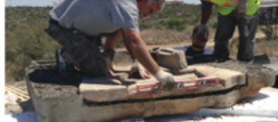
8. Set weir level left to right; draindown feature included.
